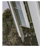
I - POWDER COATED METAL FRAMED WINDOWS DULUX FLAT WHITE POWDERCOAT PERRY PARK - CANDALPAS ASSOCIATES
